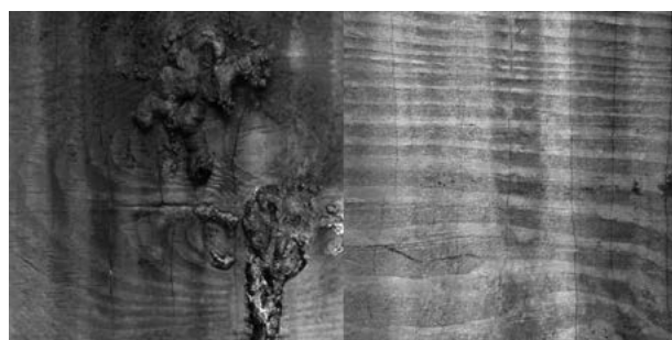
Fig 10. Views of treated pine timber specimen after tests with heat sources of 10 kW/m 2
