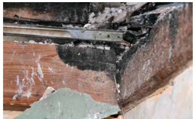
Ryc. 25, 26. Widok śladów ognia w źródle (fot. Tomasz Wiśniewski) Fig. 25, 26. Picture showing traces of fire in the ignition source (photos by Tomasz Wiśniewski)
