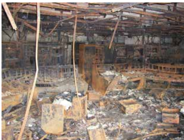
Rycina 11. Skutki pożaru w nastawni w elektrowni Figure 11. The effects of a fire in the power plant's control room
